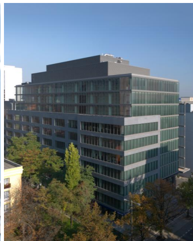
Saski Crescent, Warsaw
